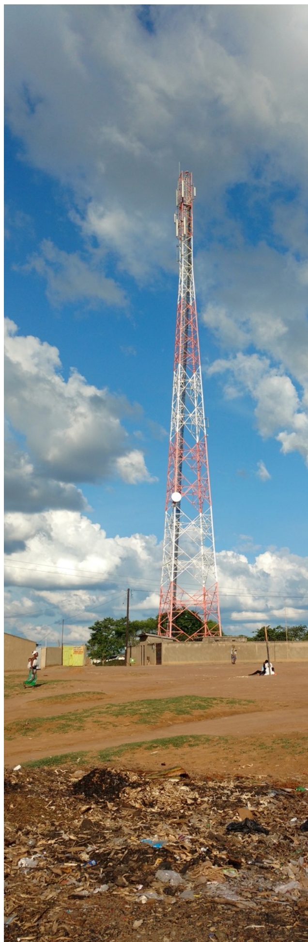
NAKIVALE CELL TOWER IN BASE CAMP
